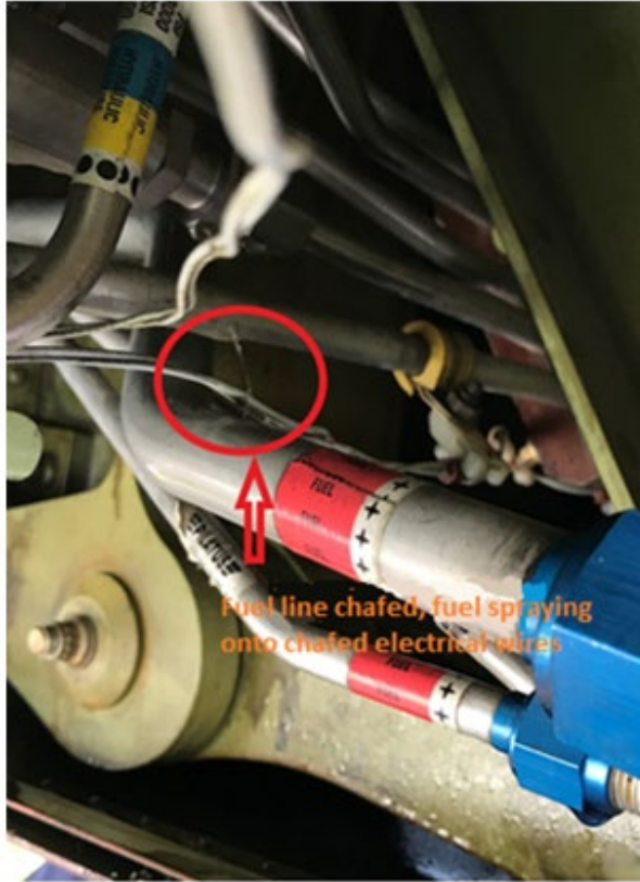
Picture 1 – Fuel stream from the chafe on the fuel line
