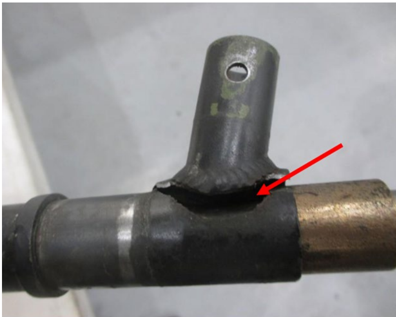
Figure 2 – Failure at weld
