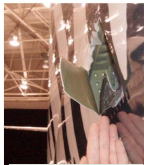
Figure E2: Photo of Skin Failure Following Ground Handling Damage (photo of 12 in. by 6 in. damage taken after flight depressurization incident)
