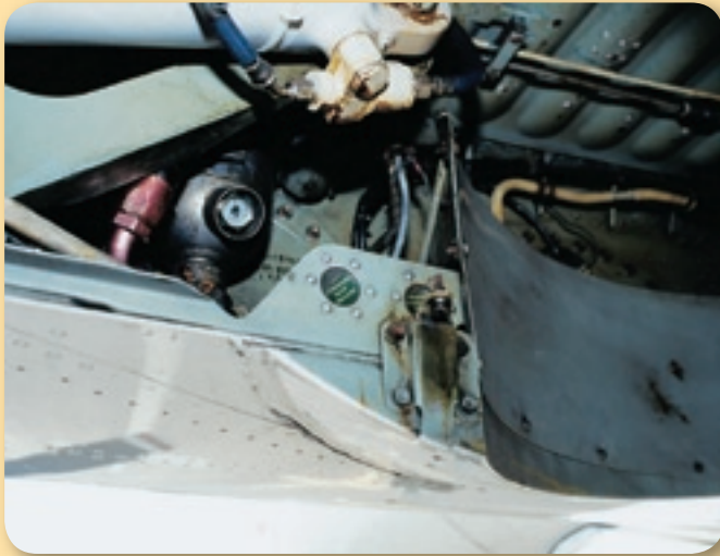
British Aerospace Jetstream Series 3200 engine compartment fire protection system.
