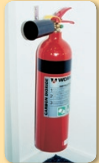
Significantly larger quantities of carbon dioxide extinguishing agent are required to put a fire out than is the case with halons.
