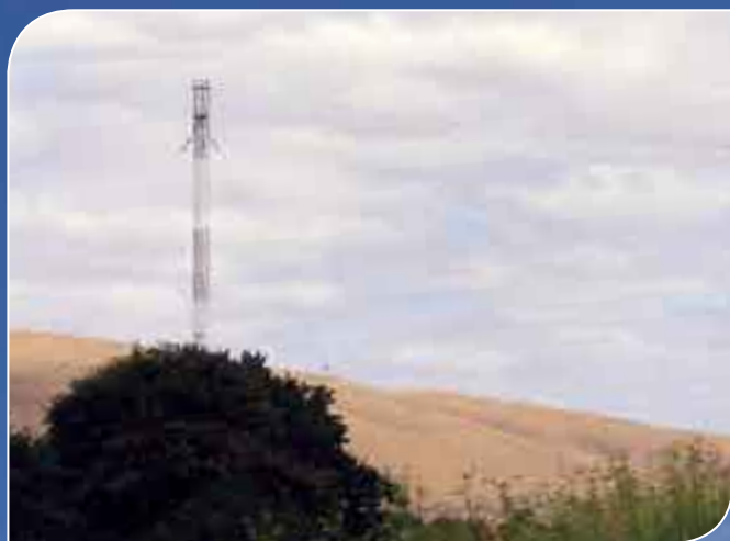
This latticework structure is easily seen in this situation, but note the guy wires and connecting wire heading off to the right.
